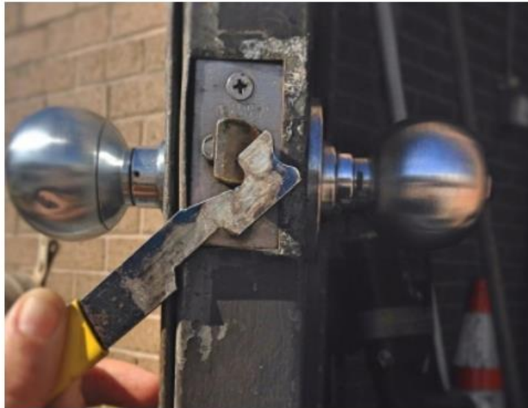
Figure 72. How a Shove-it Tool Bypasses a Latch
