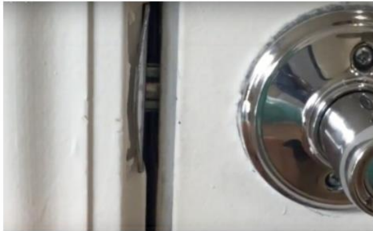
Figure 71. Shim Exploitable Door
